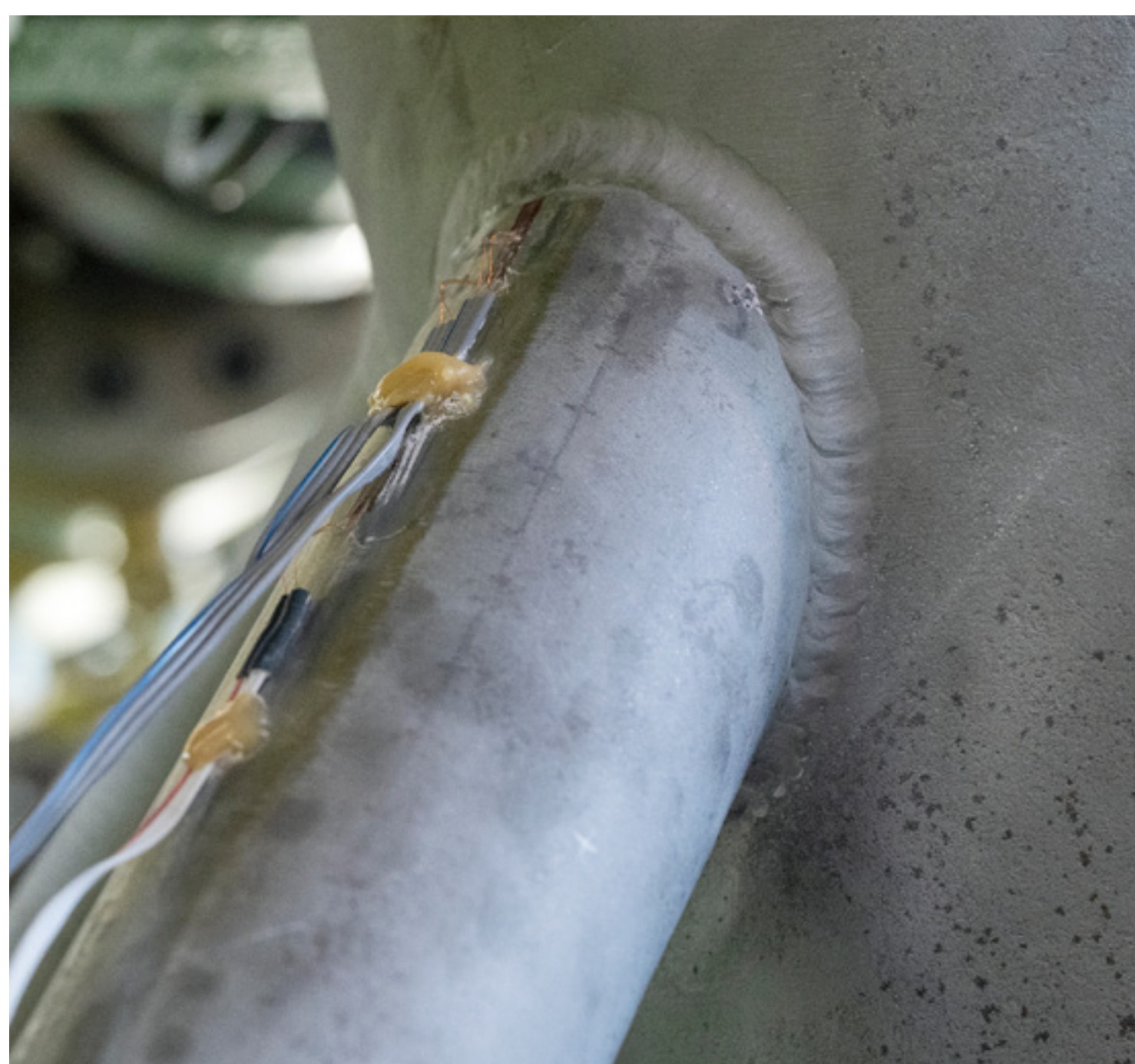
Particular focus: The weld seams of the supporting structures.
