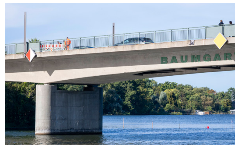
In 2025, the behavior of the prestressing wires under various traffic loads was examined on a heavily used bridge near Werder.
