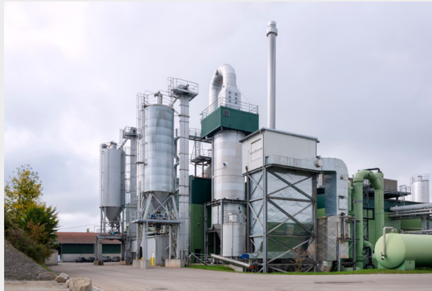
The facility for phosphorus recovery in Altenstadt, Bavaria.
